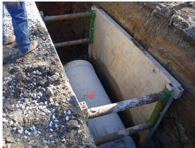
Lake Ridge Terrace Replacement
