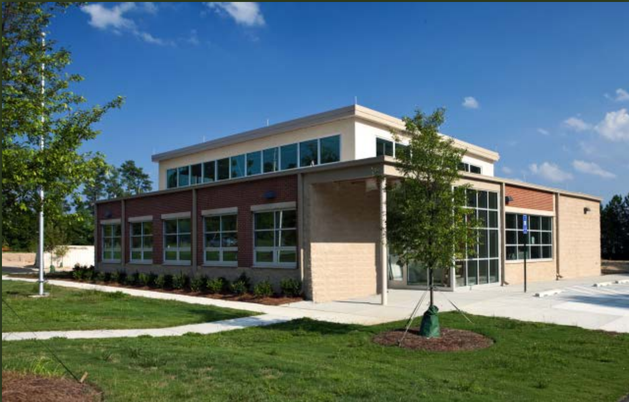
Kitchen facilities relocation and expansion
