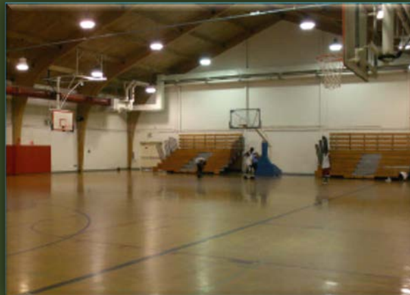
Floor refinishing/carpet replacement
